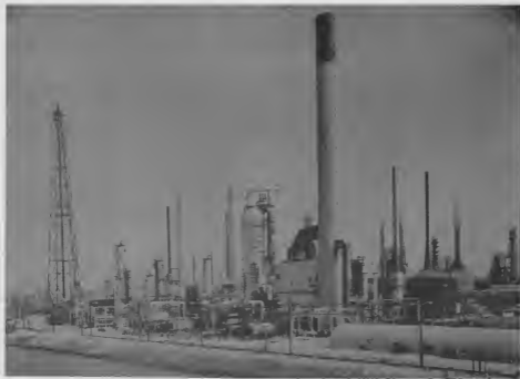
View of Hydrodesulfurization Complex, from the road. Vista di Planta Dasulfurador for di rif.
